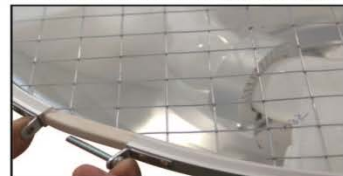
Unscrew the screws which on the Electrical Box cover with screwdriver.
