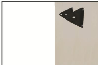
Installed stator plate lighting on the wall of the tunnel or bridge and tightened stator by screw.
