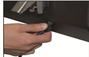
Tightening the waterproof of the connections which back to the fixture.
